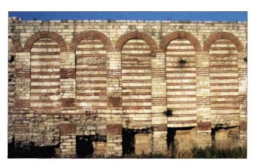
The Theodosian walls were constructed using stone and brick. In this detail of the sea wall on the Sea of Marmara both materials can be seen. Brick was used more sparingly than stone.
