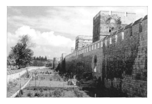
In this section just south of the Topkapi Gate we see good examples of the towers of the outer wall. One is semicircular, the other square. Both are very small compared with the towers of the inner wall behind them.The photograph was taken in 1996, since when this area has been landscaped.
