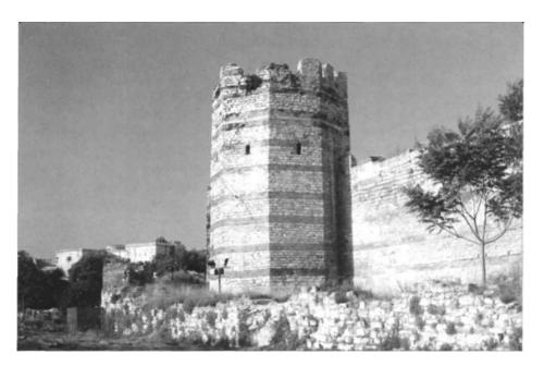
The octagonal tower just to the south of the Golden Gate, which is visible in the distance. The use of alternate layers of brick and stone is well shown.
